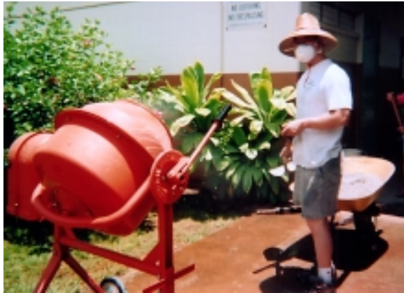
Wayne Kim spent the whole day mixing cement for the walkways.
