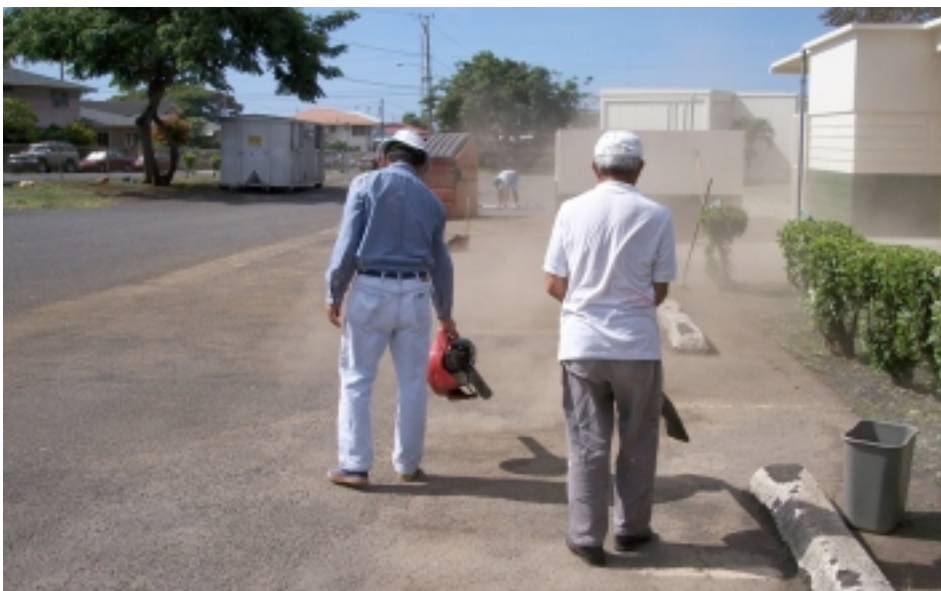
Sunny Young and Dan Takamatsu blowing away loose gravel and dirt.
